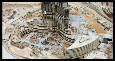
Burj Khalifa utilized a record-breaking 430,000 cubic yds. (330,000 m<sup>3</sup>) of concrete; 42,990 tons (39,000 metric tons) of steel reinforcement; 1.1 million sq. ft. (103,000 m<sup>2</sup>) of glass; and 167,000 sq. ft. (15,500 m<sup>2</sup>) of embossed stainless steel. The tower took 22 million man-hours to build.
